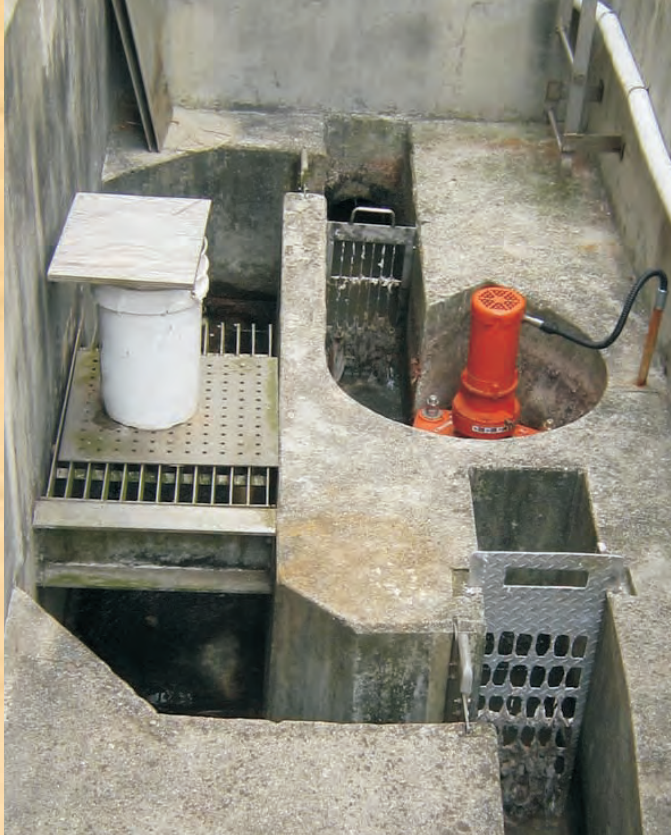
Using Existing Channel Installed GRIND HOG™ 10L
