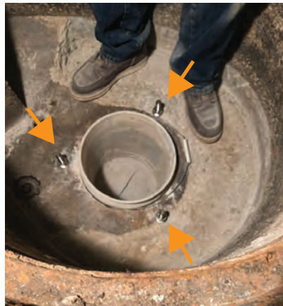
New Anchor Bolts Installed
