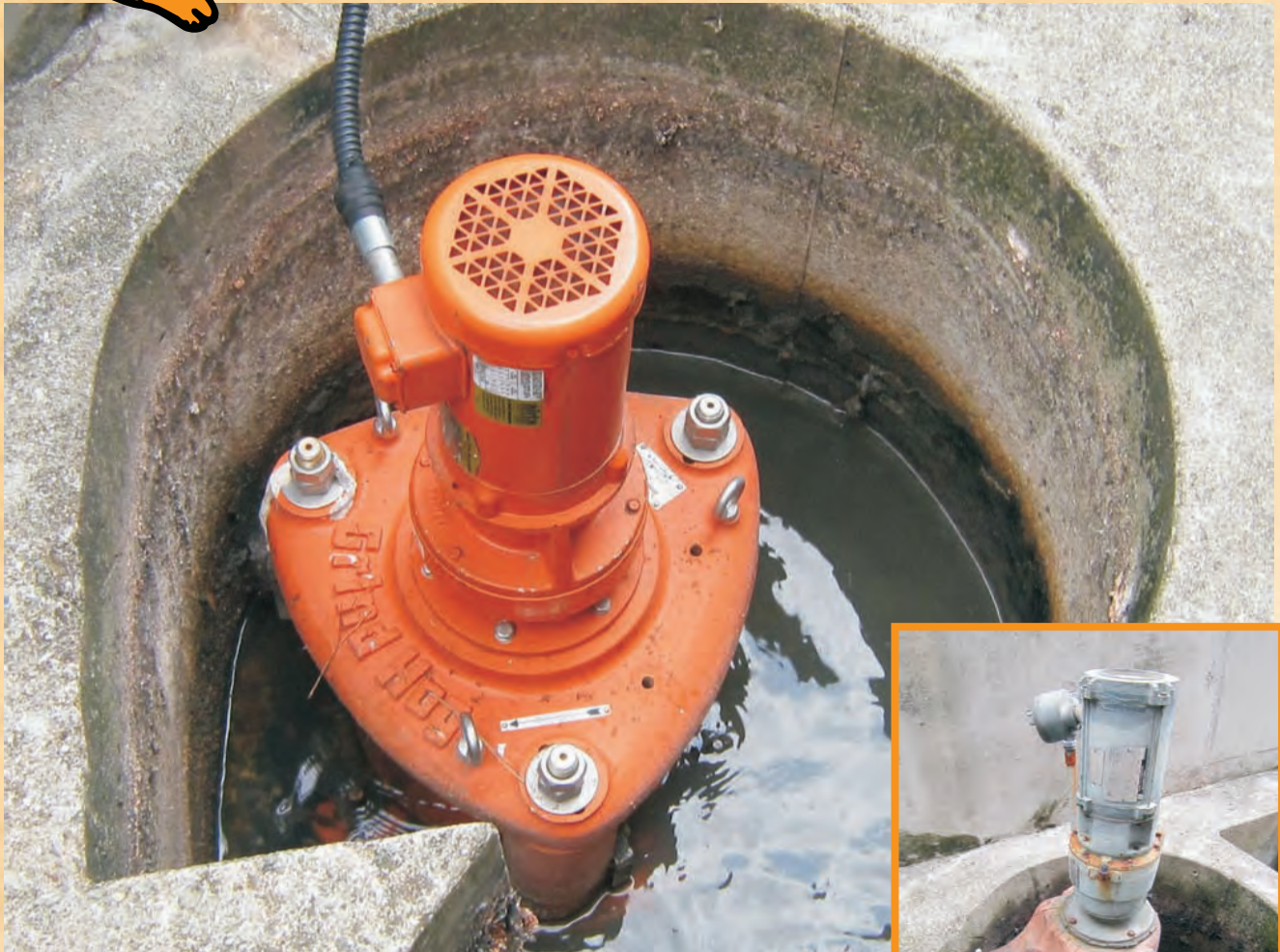
GRIND HOG™ 10L Retrofitting Chicago Pump 10C
