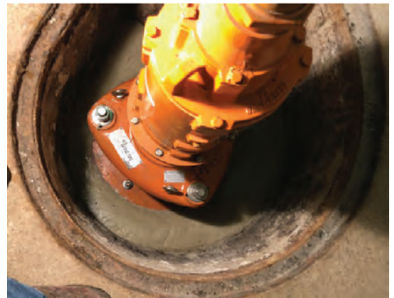
Grind Hog 10LSX Installed
