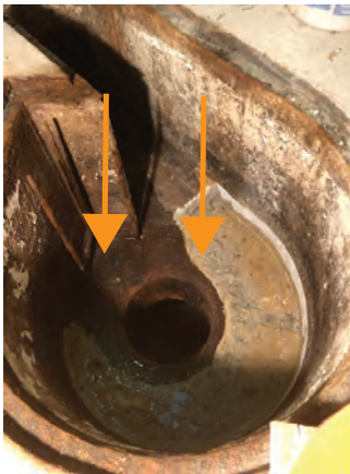
Existing Anchor Bolts Removed
