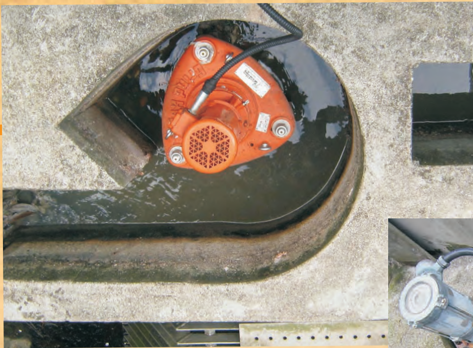
Using Existing Channel Installed GRIND HOG™ 10L
